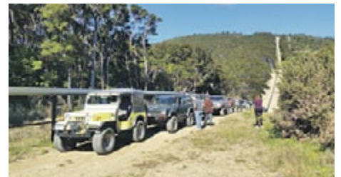
Transporting and installing sandbags along the predator-free fence at the Brook Waimārama Bird Sanctuary.
